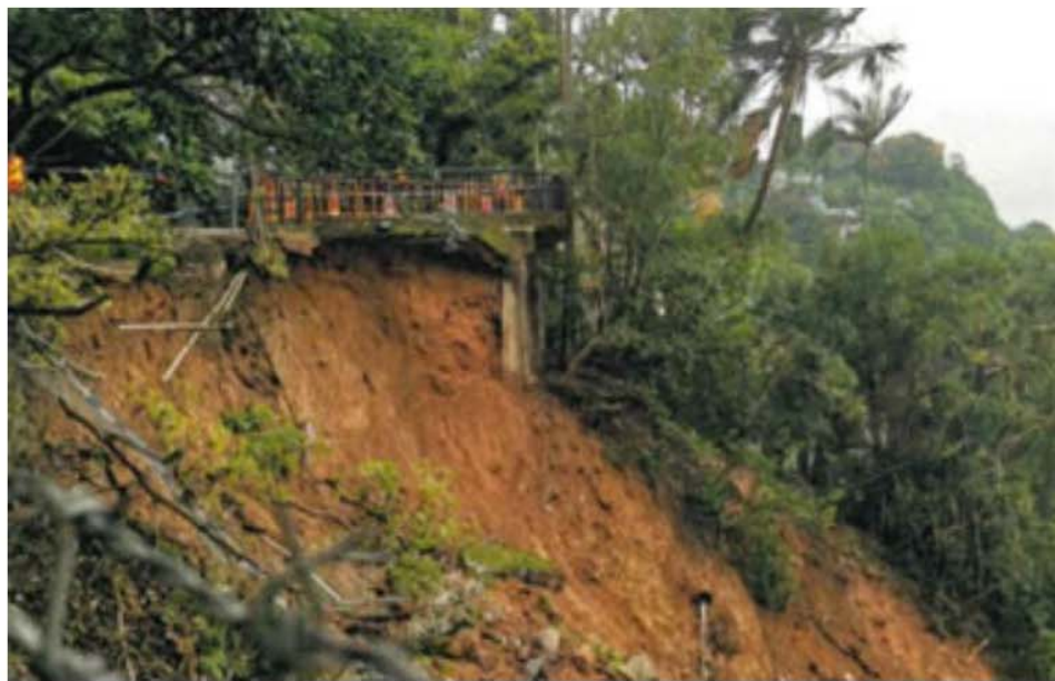
Landslide Slope near Peel Rise
